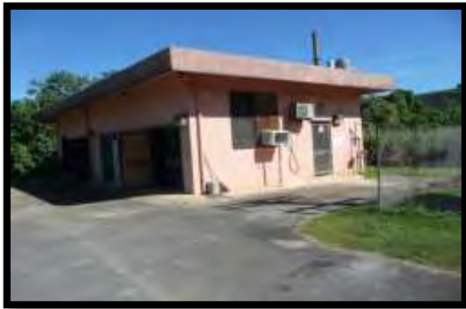
Photo 3.14-3. Maui Well #2 Pump
